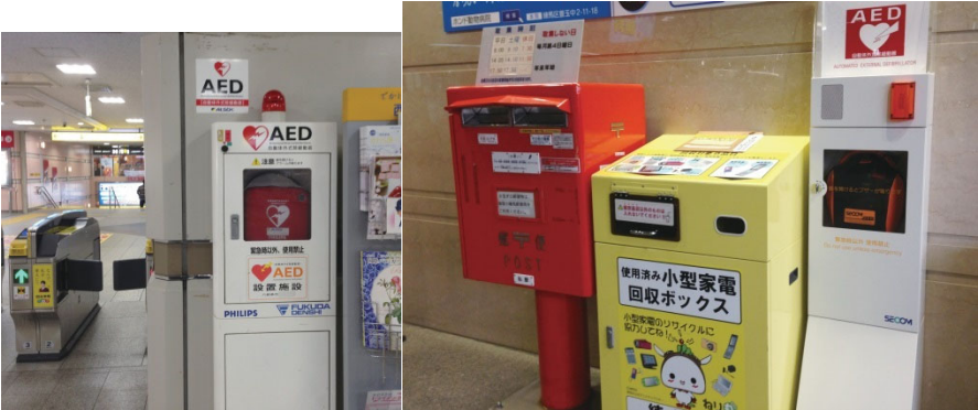
Fig. 6.7 Examples of Installed AED Boxes (Ministry of Health, Labor and Welfare, 2015)
